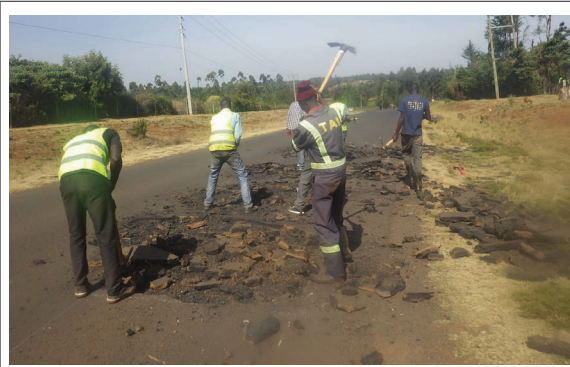
Removal of Cut Asphalt
