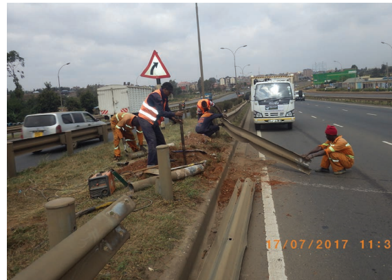
Damaged guardrail removal
