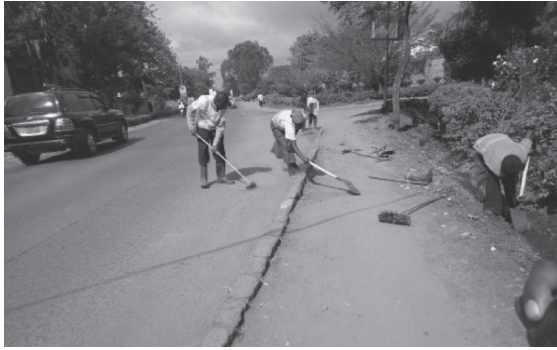
De-siltation of drainage and cleaning of carriageway
