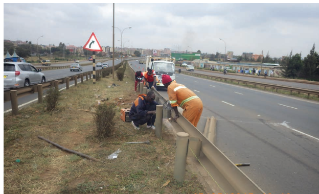
Fixing of straightened beam
