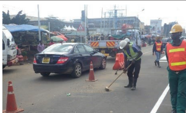
Cleaning of Road Surface
