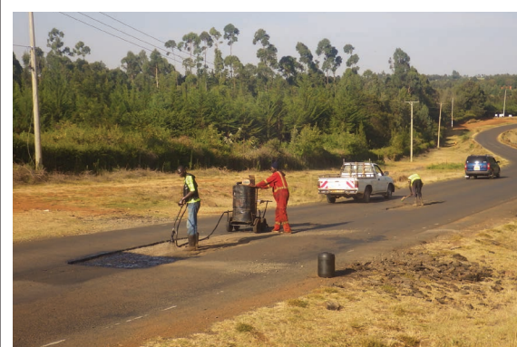
Spraying of Tack Coat
