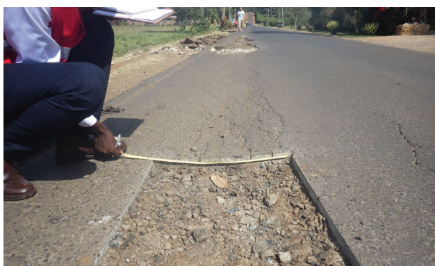
Measurement of Pothole
